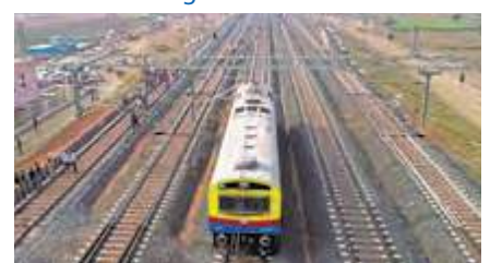
Dedicated Freight Corridor
